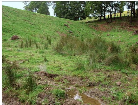
Earthen dam seepage
