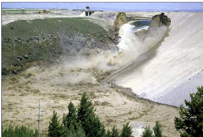
Failure of Teton Dam (Idaho) from seepage (1976)
